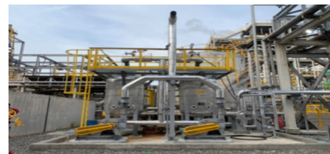
Improvement of TDI air pollution control facility (KRW 1.1 billion investment)
