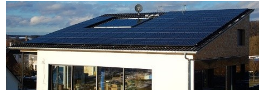
Solar modules installed on households in Augsburg, Germany by Q CELLS
